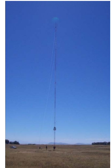
80m monitoring mast at Hopefield site
